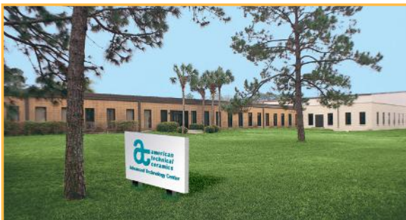
▲ Advanced Technology Center, Manufacturing Facility, Jacksonville, Florida
